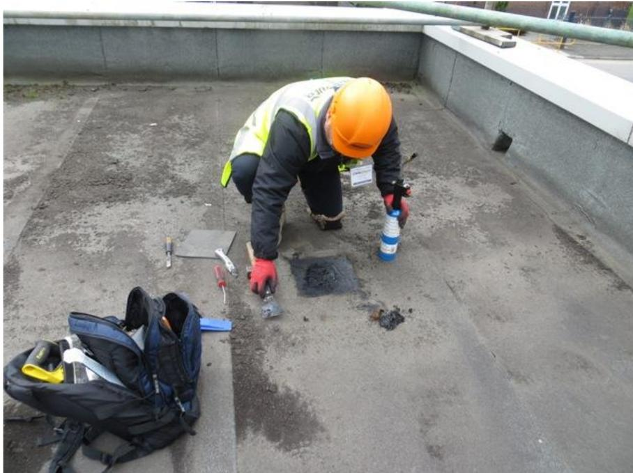
*Figure 5: Staff from Bauder checking waterproof layer of the roof before deciding if the roof was suitable for a green roof.*
